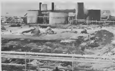
Preparation of Hydrogen Plants site north of Powerhouse No. 1 in June 1969.
